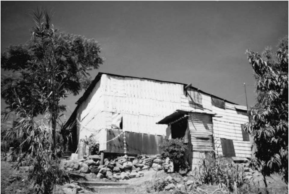
Plate 4.1 Self-built house, informal settlement, Oaxaca City, Mexico.
