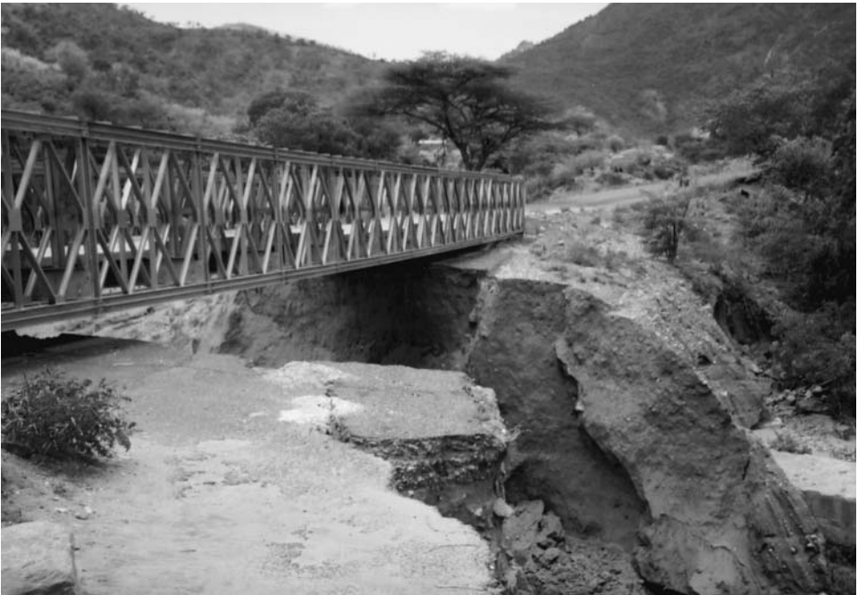
Plate 6.1 Temporary road bridge, Ortum, Kenya.
